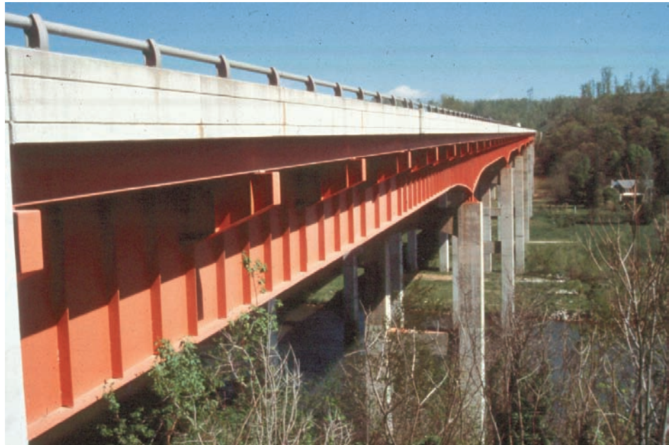
Figure 8.3.13 Flexural Zone on a Two Girder Bridge
