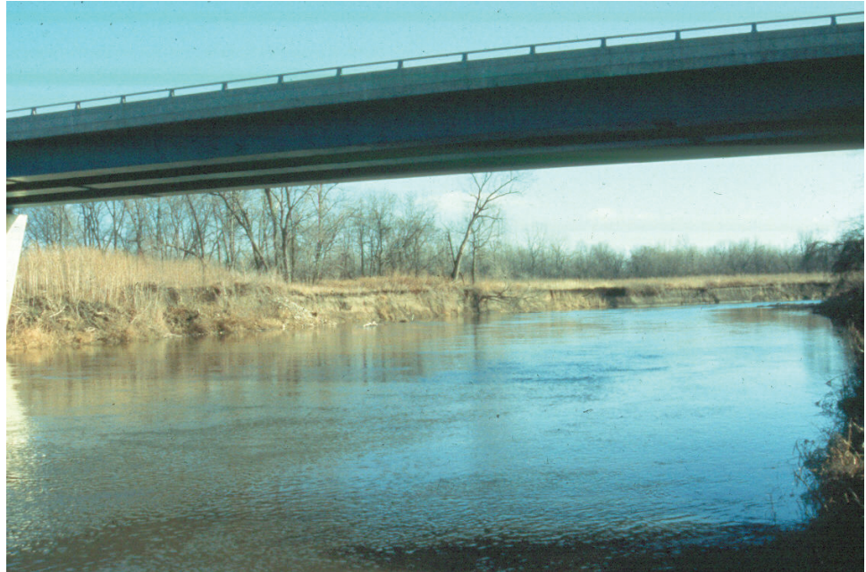
Figure 8.5.1 Simple Span Box Girder Bridge
