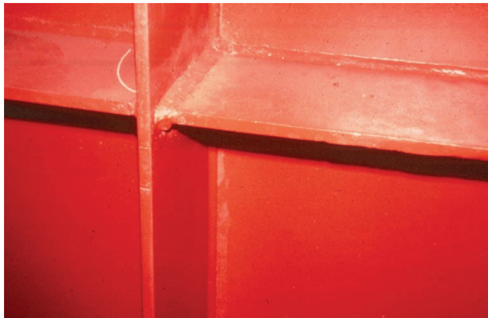
Figure 8.3.21 Intersecting Welds
