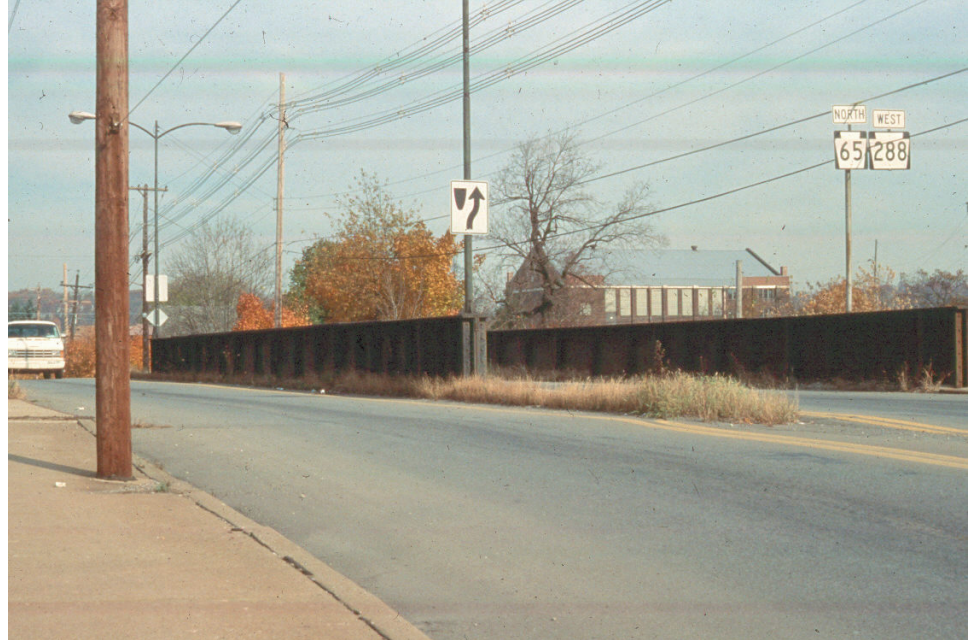
Figure 8.3.4 Through Girder Bridge with Three Girders
