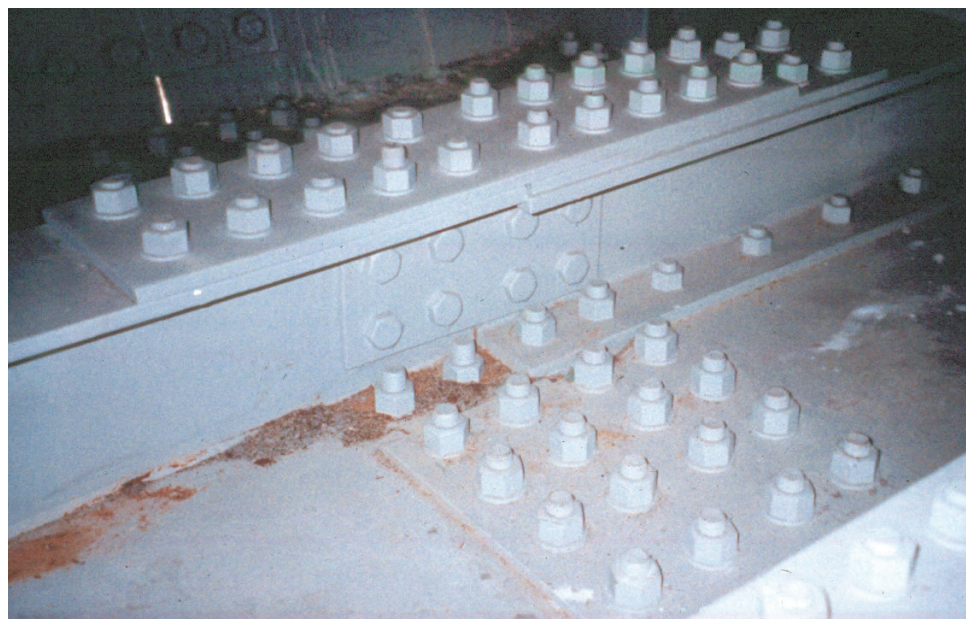
Figure 8.5.12 Field Splice
