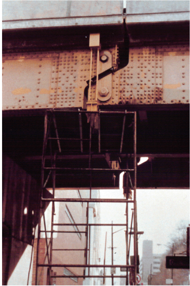
Figure 8.4.18 Alternate Hanger Link Retaining System
