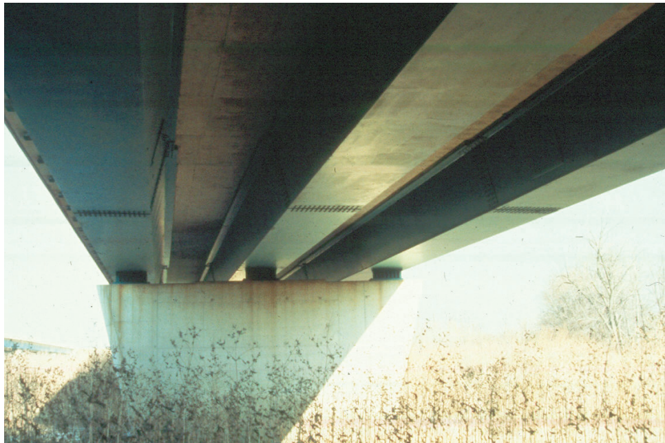
Figure 8.5.15 Redundant Box Girder Bridge
