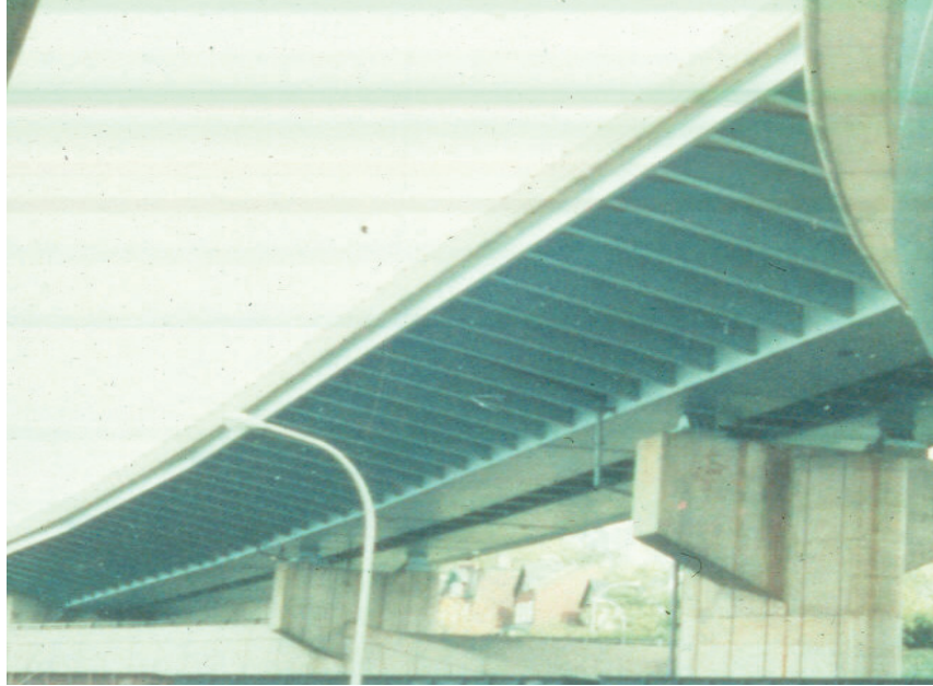
Figure 8.5.14 Non-redundant Box Girder Bridge
