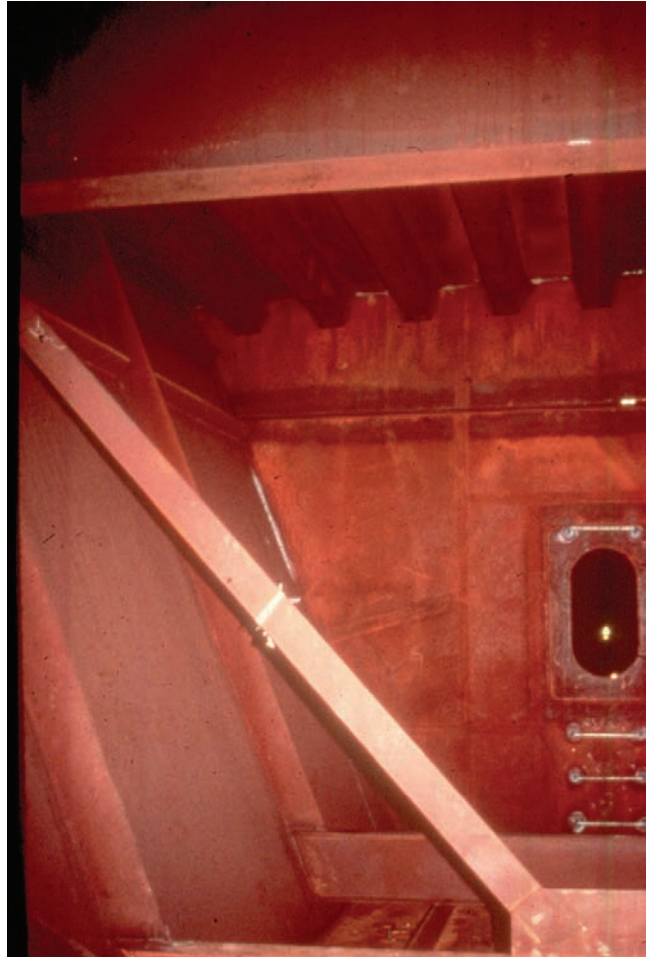
Figure 8.5.5 Diaphragms – K Bracing and Plate
