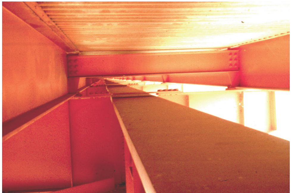
Figure 8.3.29 Tie Plate for Cantilever Floorbeam
