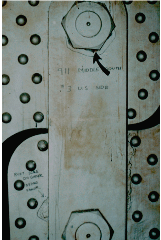
Figure 8.4.6 Threaded Pin with Retaining Nut
