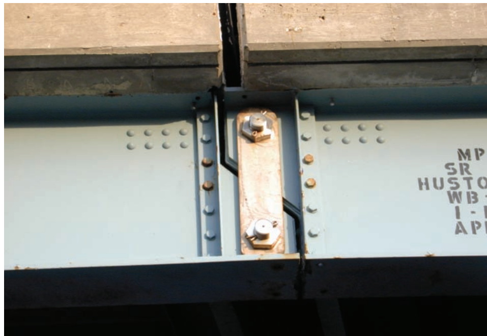
Figure 8.4.25 Stainless Steel Pin and Hanger Assembly
