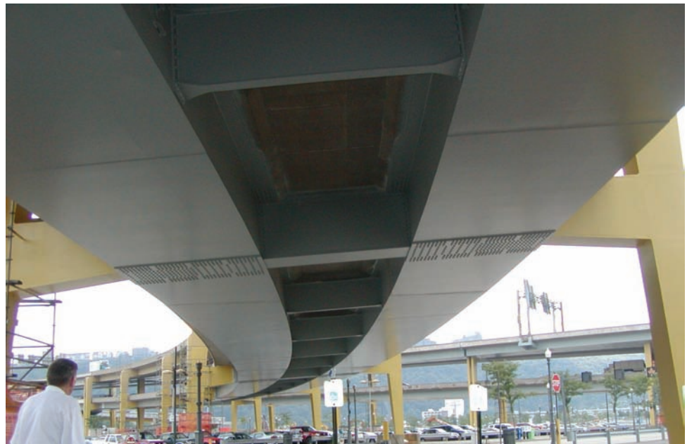
Figure 8.5.4 Spread Box Girders
