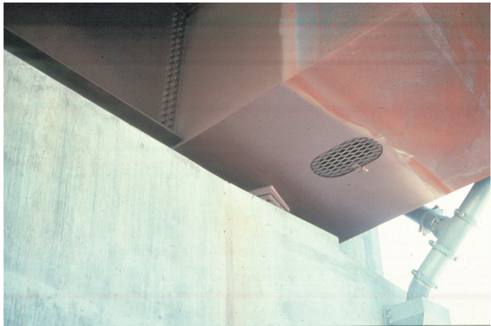
Figure 8.5.10 Box Girder Shear Zone
