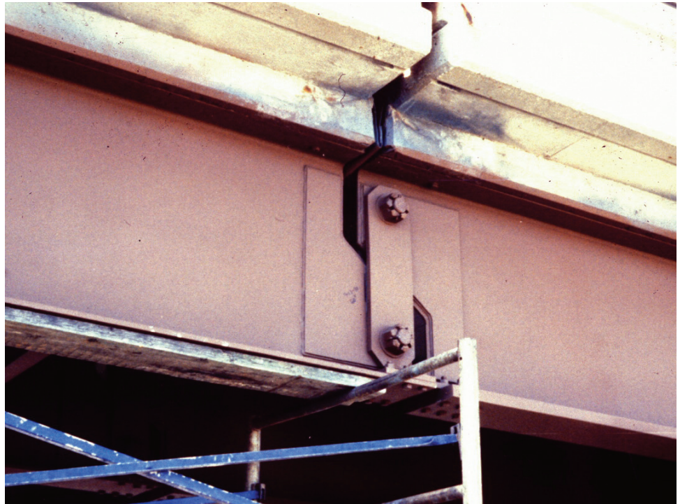
Figure 8.4.1 Typical Pin and Hanger Assembly
