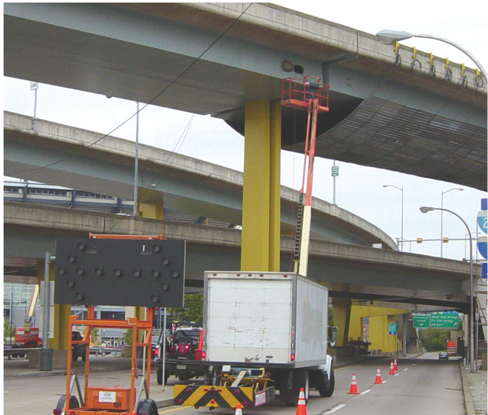
Figure 8.5.7 Box Girder Access Door
