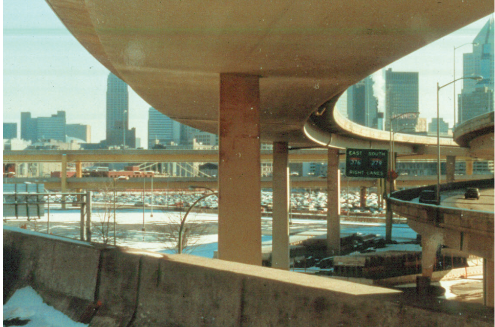
Figure 8.5.3 Box Girders With Cantilevered Supports for Deck
